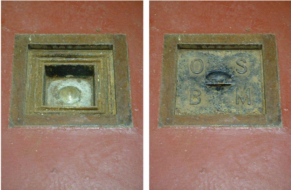
Ordnance Datum Newlyn: The brass bolt marker (L) sits under a cover (R)
