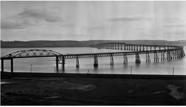
1 The Tay Bridge just after completion, showing the centre or 'high girders' section needed to allow passage of high masted sailing ships upstream along the river to Perth (clearance was about eighty-eight feet at high tide). Some finishing work was still being performed on the bridge, judging by the staging and ladders seen at various points
