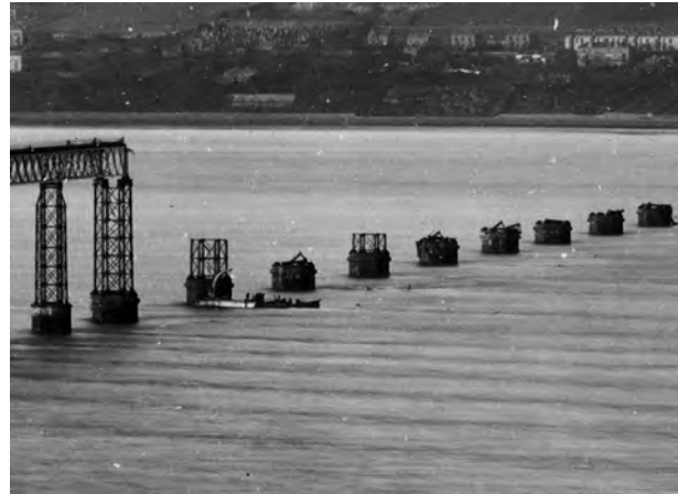
4 Closeup of the join between the low and high sections of the bridge showing partly intact tiers on two piers. The boat in the foreground is searching for survivors in the girders, which are just visible in front of the third fallen pier, poking above the waterline. Numerous tie bar breaks can be seen in the centre of the last standing tower
