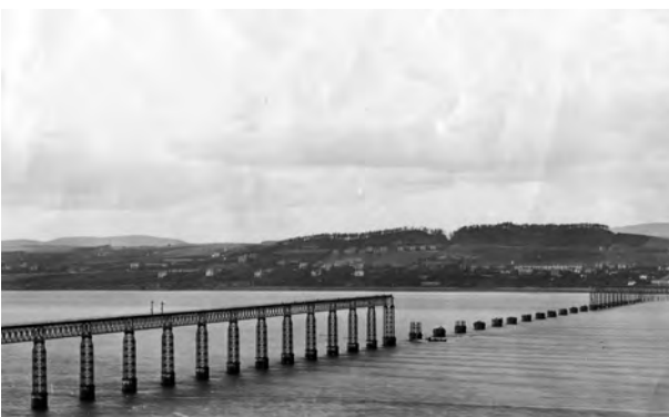
3 Long shot of the collapsed high girders section of the bridge, with twelve pier platforms almost completely swept off their high towers
